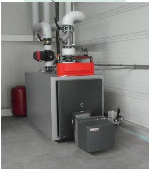
Example of a boiler for central heating of 2 sections.
